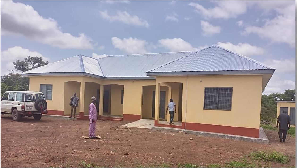
Figure 1: Constructed 1 No. CHPs Compound at Jakpumba
