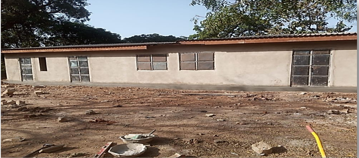
Figure 6: Ongoing Rehabilitation of 1 No. 3-Unit Classroom Block at Dakpam
